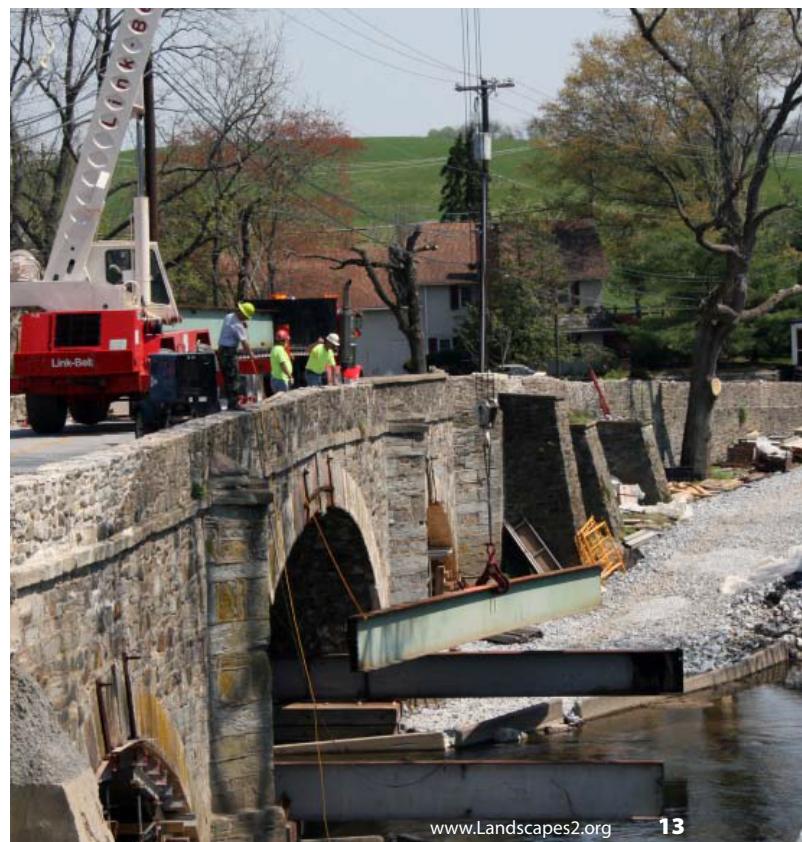
Historic Copes Bridge on Strasburg Road underwent major restoration.
