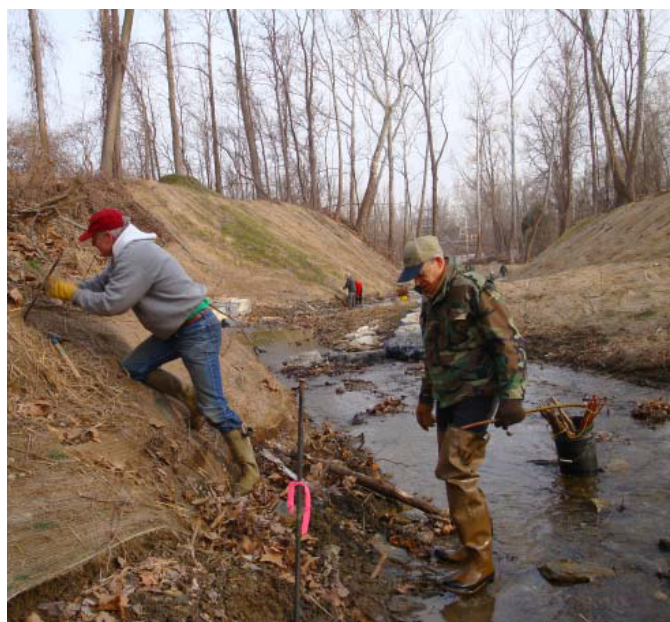
Volunteers installing plants along streambank to protect against stormwater erosion.
