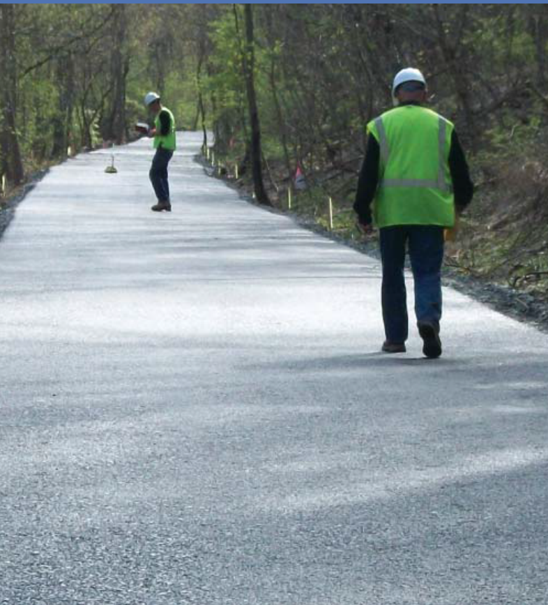
Significant progress occurred on constructing the Chester Valley Trail during 2009.
