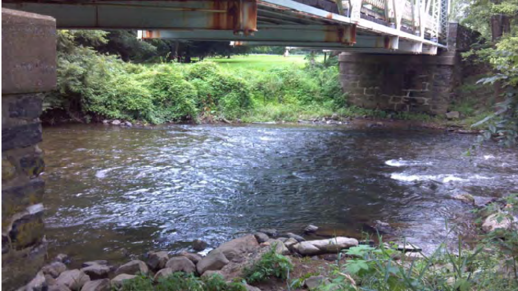
Plate 7. The modern bridge crossing is reportedly at the same location as the 1777 ford. View to the east under the bridge, showing the east branch of the Brandywine.
