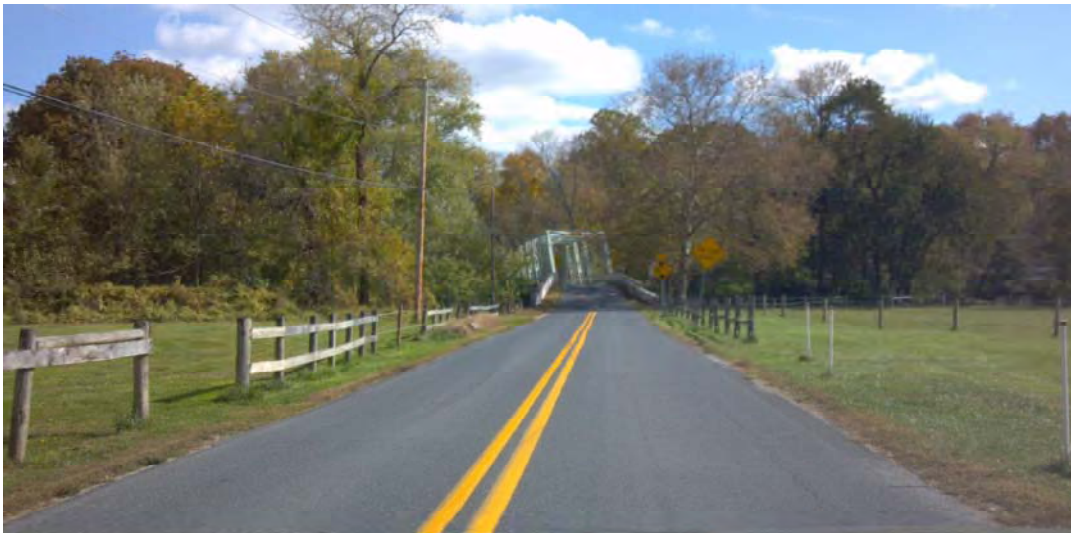
Plate 6. View to the east along Allerton Road, looking at modern bridge crossing at Jefferis Ford.
