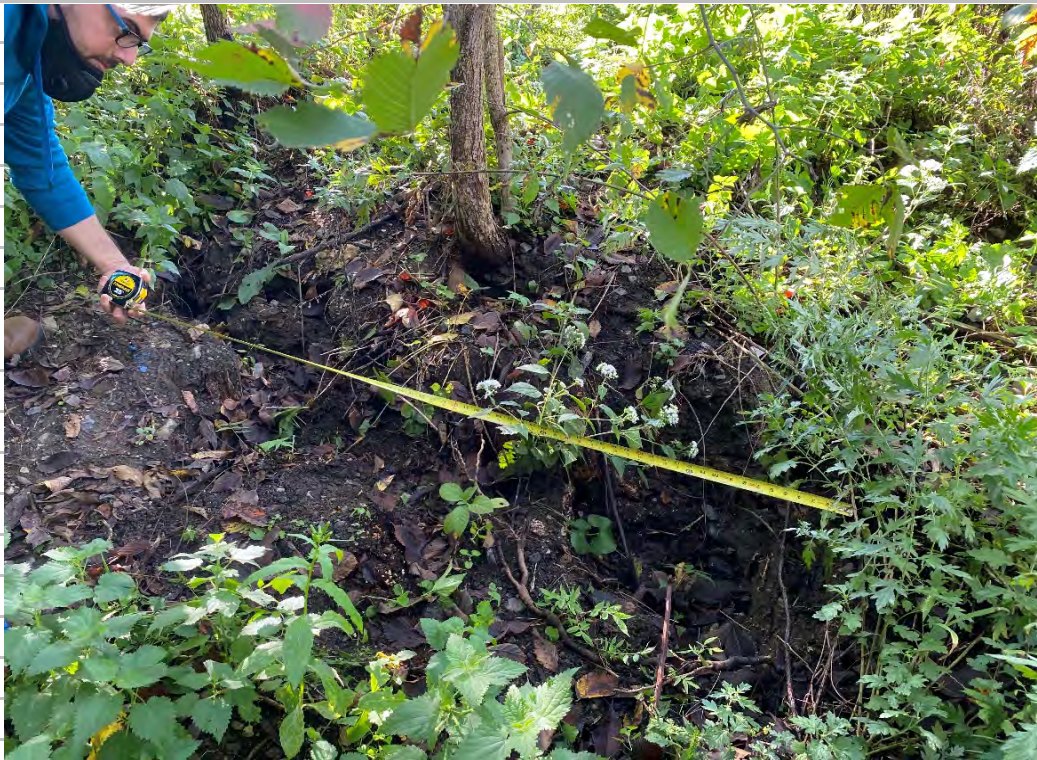
Photo 3. Potential (old) sinkhole just outside of the R.O.W.
