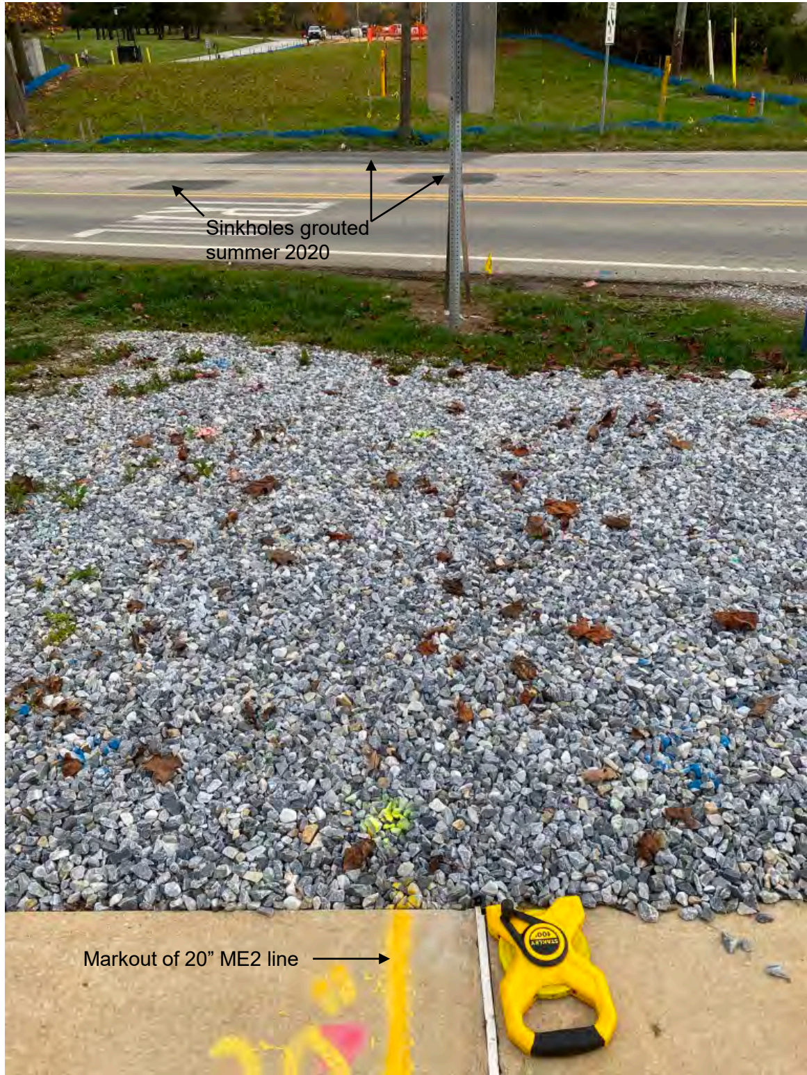
Photo 7. Sinkholes repaired along Lincoln Highway.
