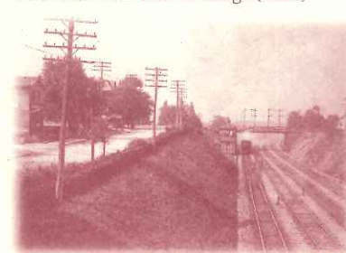
View west from Station Bridge (1905)
