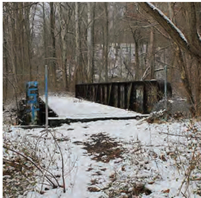
Rail Bridge crosses Marsh Creek north of Dorlan's Mill Road
