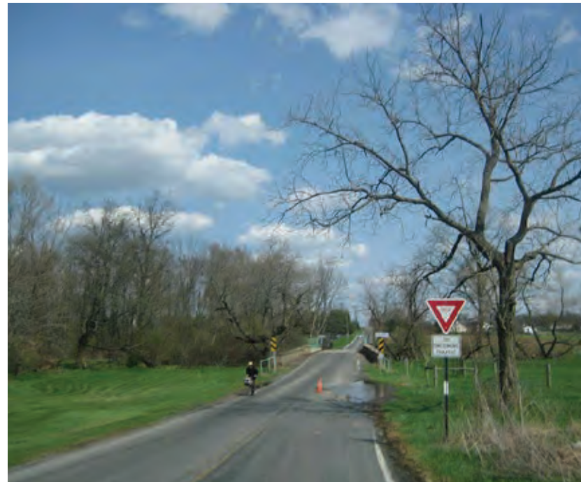
Narrow roads in Honey Brook typically lack shoulders.
