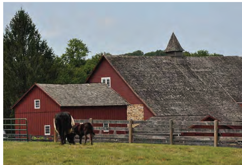
Springton Manor County Park equestrian barn.
